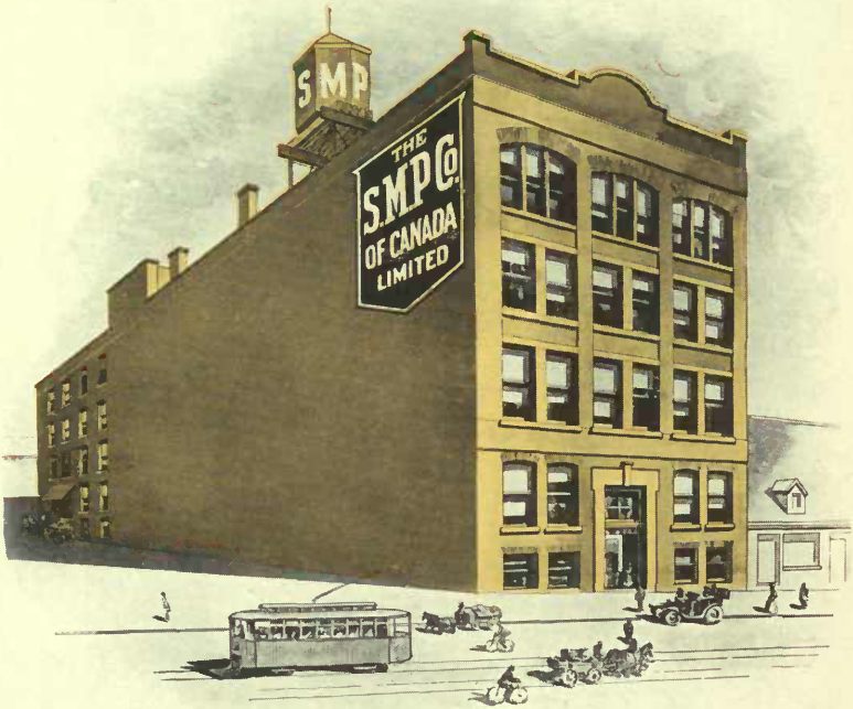
Montreal Office and Warehouse, St. Antoine Street, Montreal.
